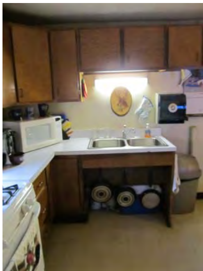
Units that have been modified for handicap accessibility include knee clearance space under the sink
