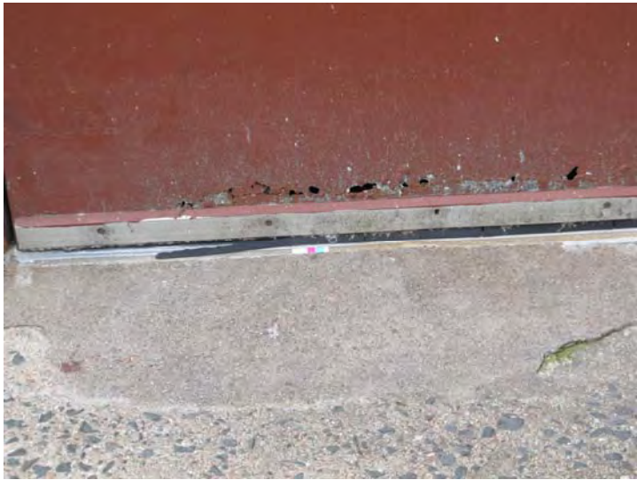
Rust damage noted on some exterior unit entry doors at handicap accessible units
