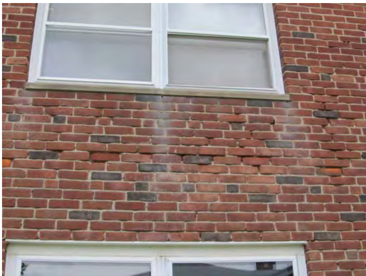
Brick veneer exhibits areas of wear/mortar loss at various locations – Building 3 exhibits most severe conditions
