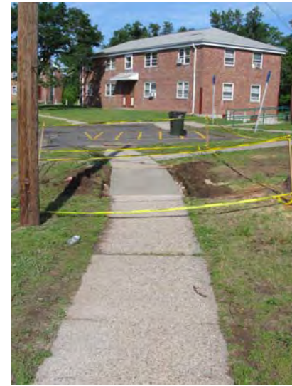
Sectional replacement of concrete sidewalks along public roadways ongoing at time of assessment
