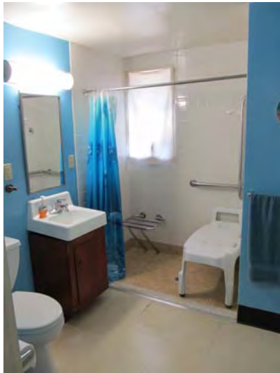
Units that have been modified for handicap accessibility include roll-in showers
