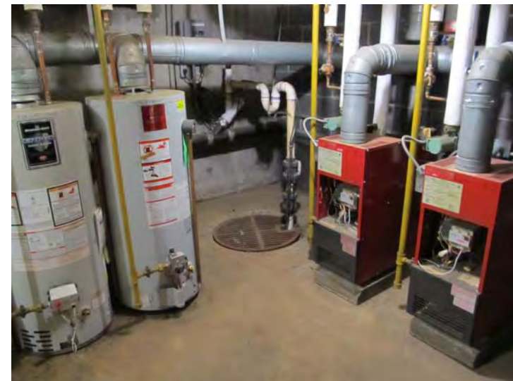
Typical heating and domestic hot water generation equipment – 1 natural gas-fired boiler per unit and 1 natural gas-fired domestic hot water tank per pair of units
