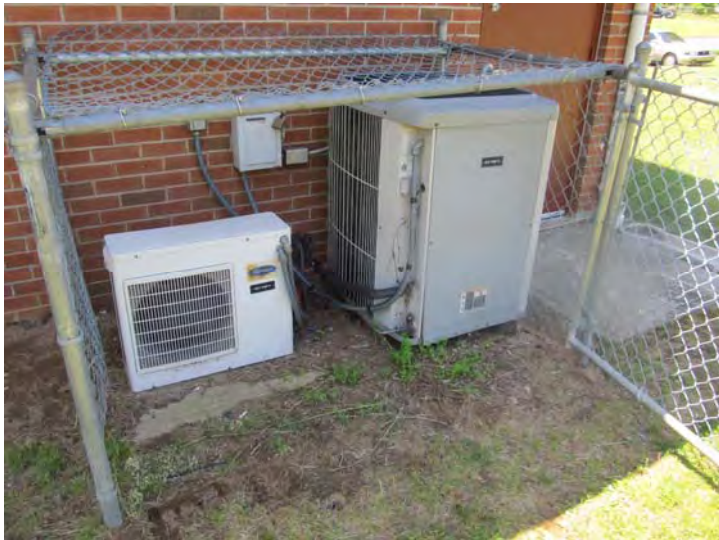
Exterior condensers for heat pump systems serving community building – No problems observed or reported
