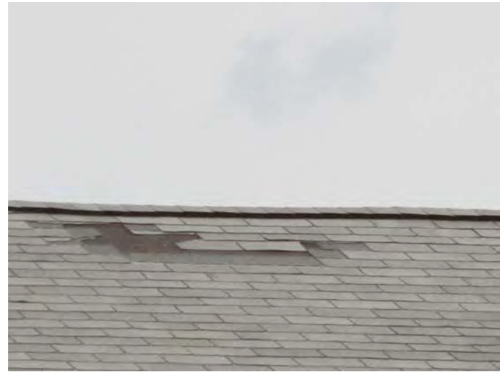
Wear and/or damage noted on roof surfaces at various locations throughout the development
